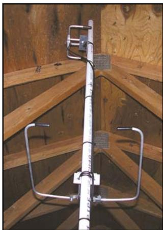
**Figure 2—My attic SQ loop installation.**
