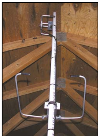
Figure 2—My attic SQ loop installation.
